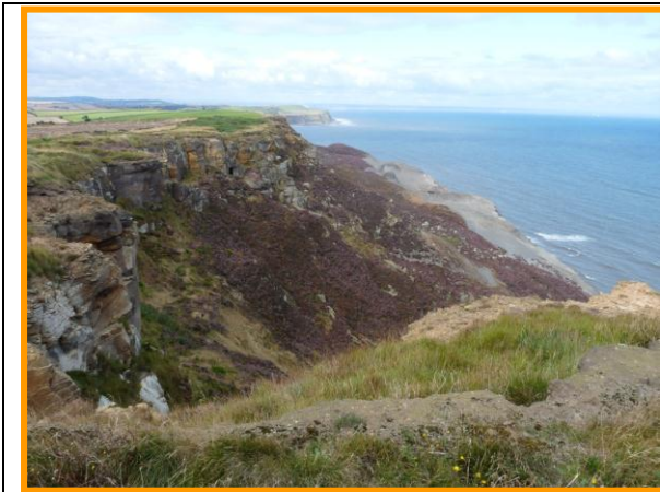
E58/4, Upper cliff has previously been quarries but is well vegetated. Lower cliff is actively retreating due to marine erosion (indicated by arrow). Upper cliff is Locally Active, lower cliff is Partly Active.
