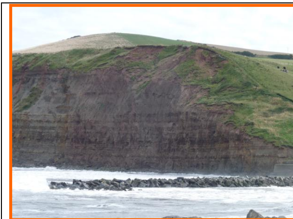
E57/7 looking southeast across the bay at Skinningrove (Partly Active)
