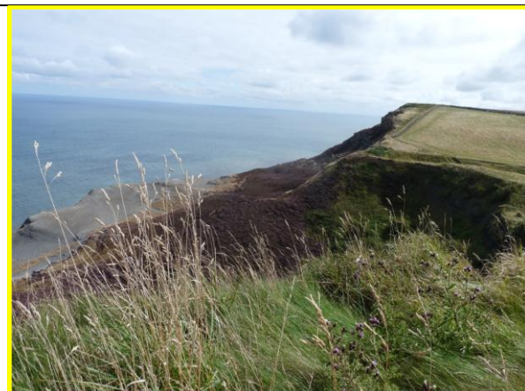
E56/5 (East) – Vegetated upper slopes and lower slopes formed of quarry waste over an active natural sea cliff.
