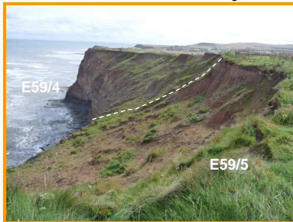
E59/5 and E59/4 Very active headscarp in till (Partly Active)
