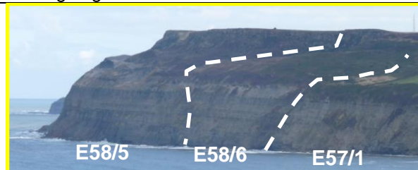
Unit 58/6, The Warren has vegetated upper slopes and lower slopes formed of quarry waste over natural cliffs (Locally Active).
