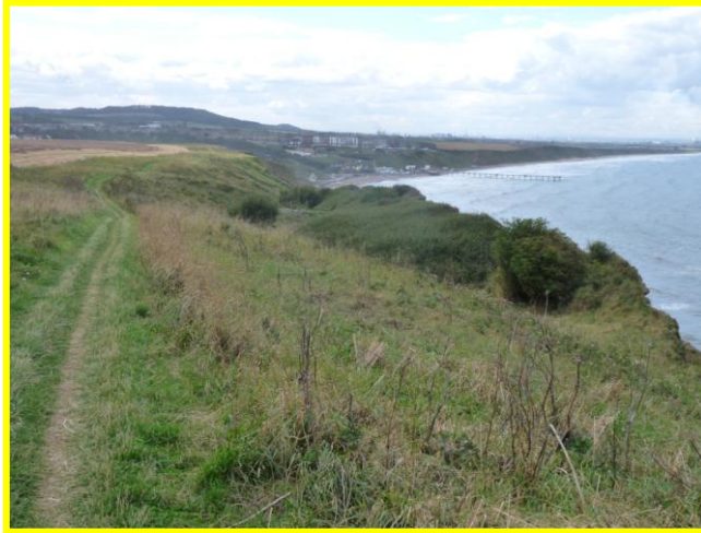
E53/2 Evidence of previous instability in the upper till section of this unit (Locally Active). Photo August 2014
