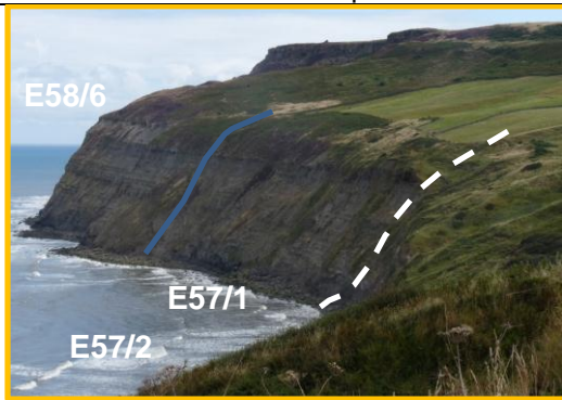
E57/1 (Locally Active) and E57/2 (Partly Active) – These units have an active and steep lower sea bedrock and a less active and well-vegetated, lower angle upper cliff. The lower angle, well vegetated part of E57/2 forms a much greater part of the cliff than at E57/1
