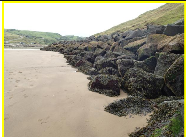
Rock armour in fair to good condition (Asset Ref No. 1221D901D0202C01)
