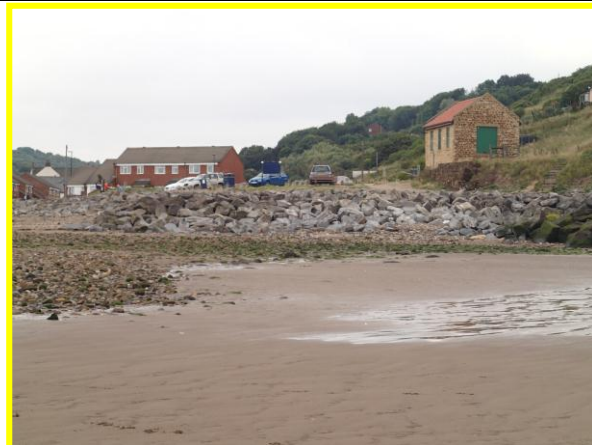
Cobble beach has accreted around the spur groyne at end of the beck (Asset Ref No. 1221D901D0202C02)
