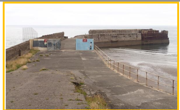
View of Jetty 24/07/2014 (Asset Ref No. 1221D901D0201C02)
