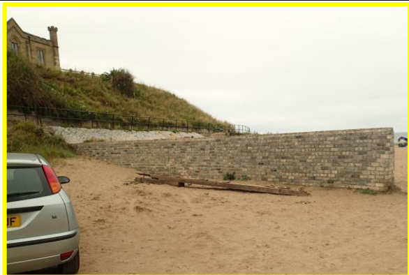
Wall enclosing fishing boat park (Asset Ref No 12221C901C0702C02)
