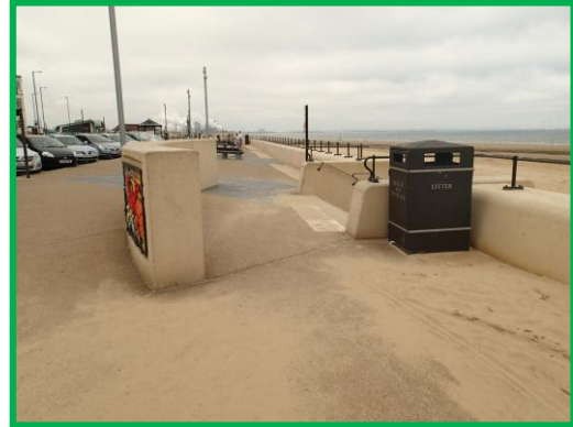
Promenade and wave wall in very good condition, Asset ref. 1221C901C0602C06
