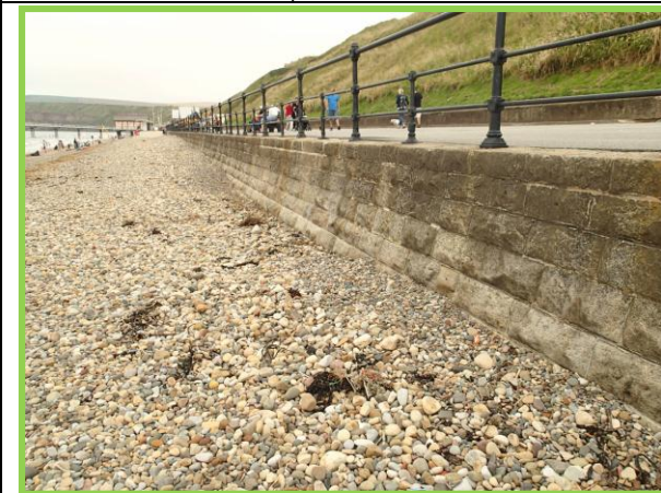
General view of wall looking south east (Asset Ref No 1221C901C0704C04)
