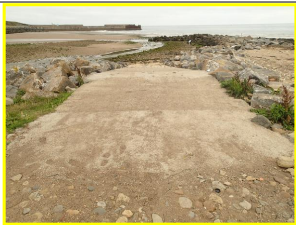
Slipway with repaired section near crest. (Asset Ref No. 1221D901D0202C05)
