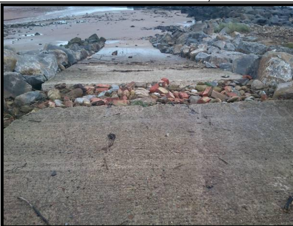
Slipway from boat park Photo from 2012. (Asset Ref No. 1221D901D0202C05)
