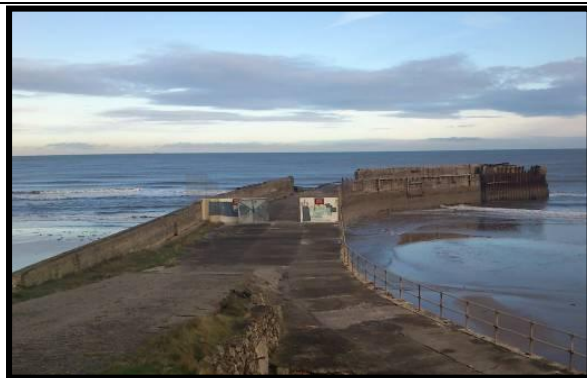
View of Jetty in 2012 (Asset Ref No. 1221D901D0201C02)
