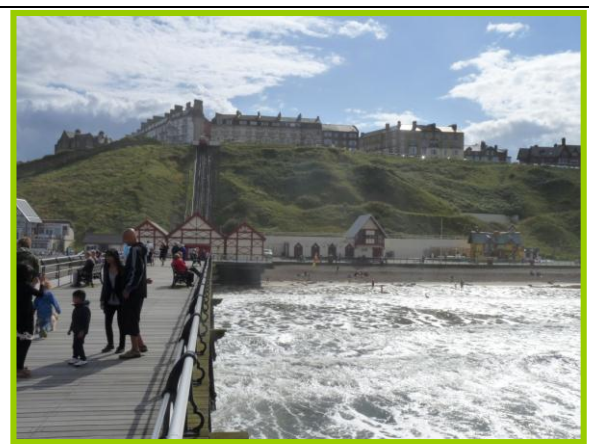
E52/3a the stabilised slopes close to the Cliff Lift (Inactive) Photo August 2014
