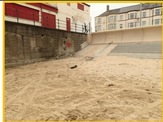
Interface between new seawall and cinema wall, Asset ref Nos. 1221C901C0602C05 & 6
