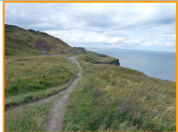
E54/2b some vegetation cover on the upper part of the cliff, looking west (Partly Active) Photo August 2014
