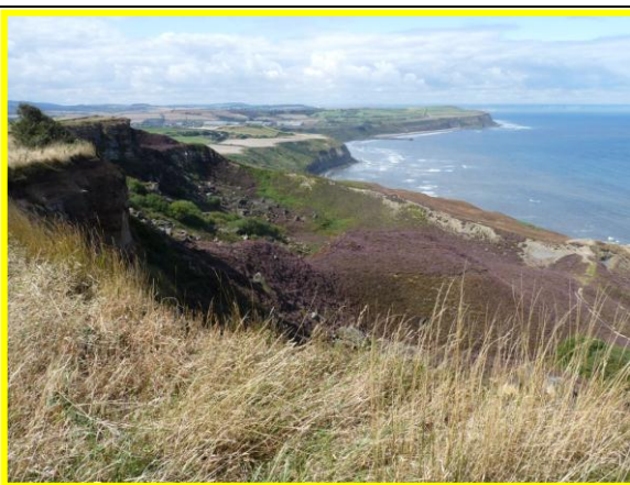
Unit 58/5 (West), Vegetated upper slopes and lower slopes formed of quarry waste over natural cliffs (Locally Active).
