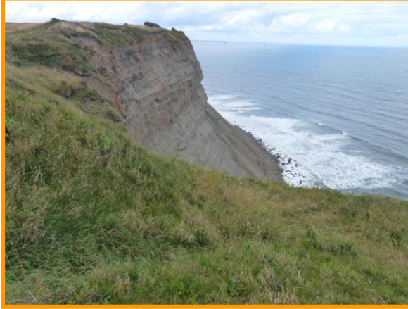
E54/4 looking northwest along Hunt Cliff showing active cliff face and debris apron (Partly Active) Photo August 2014
