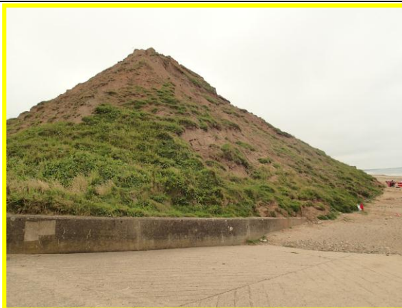
Eroding cliff (E52/4) adjacent to ramp at the north of Hazel Grove Foot, (Asset Ref No 1221C901C0703C02).
