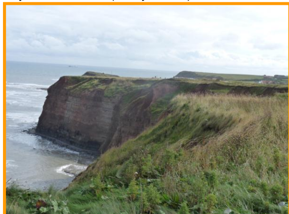
E59/3 lower cliff subject to marine erosion and cliff top actively receding (Partly Active)
