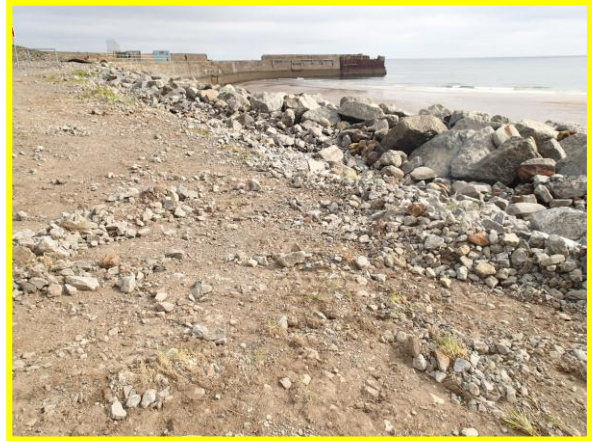
Rubble fill at crest has been reprofiled (Asset Ref No. 1221D901D0202C01)
