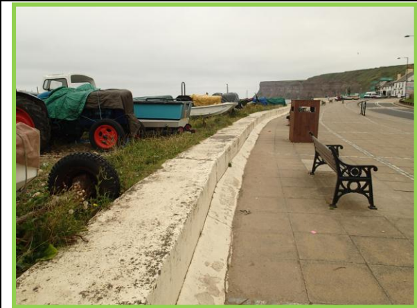
Set back rendered wall protected by shingle beach (Asset Ref No 1221C901C0704C03)
