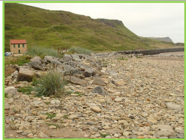
Shingle ridge photo from 24/07/2014. (Asset Ref. No 1221D901D0202C04)
