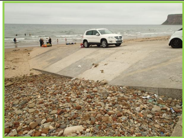
Repaired slipway at east end of Asset Ref No 1221C901C0704C03
